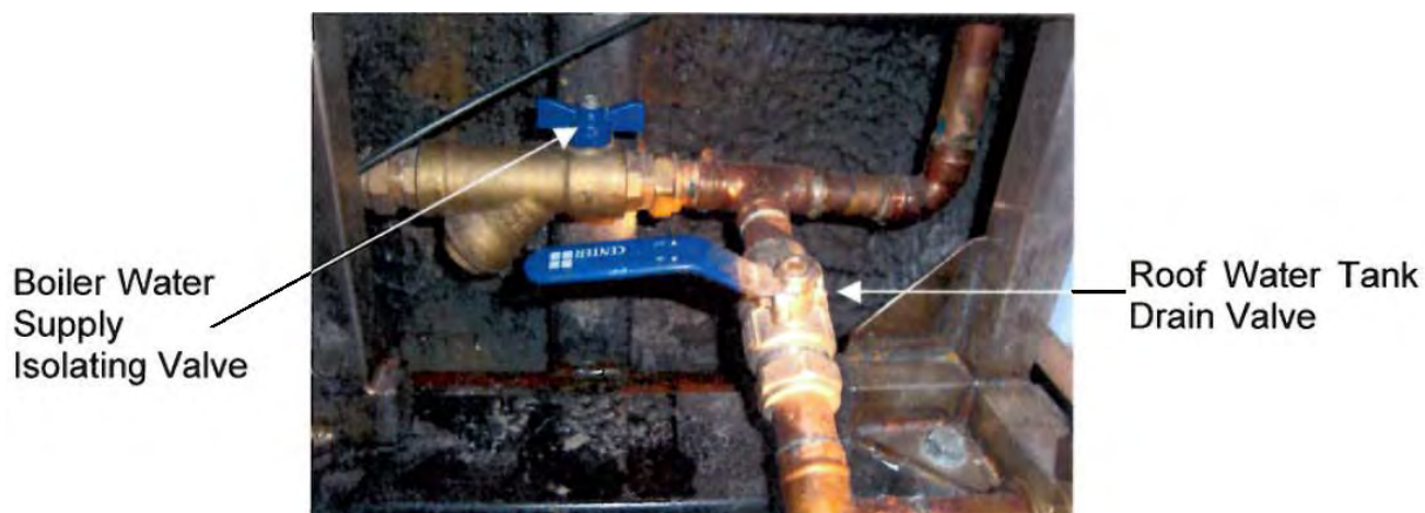
Figure 2.4: TSB Roof Tank Drain and Water Supply Isolating Valves
