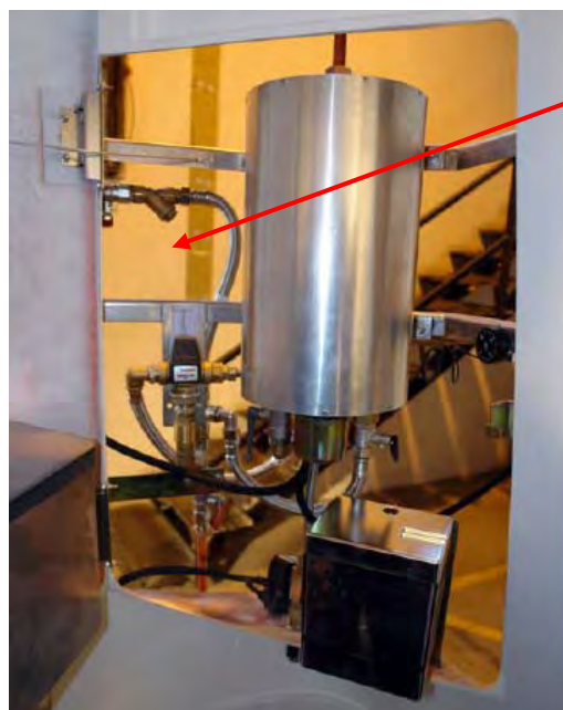
Figure 1: Water Filter Installation
