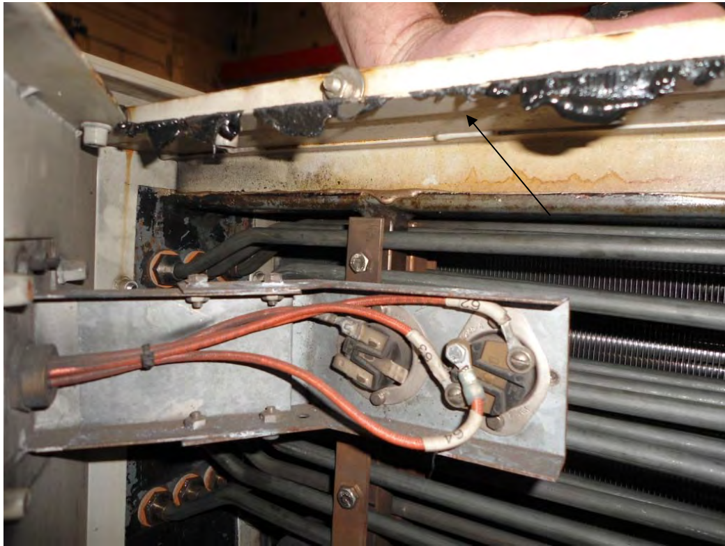
Figure 3: Typical View of Over-Temperature Thermostats in Situ
